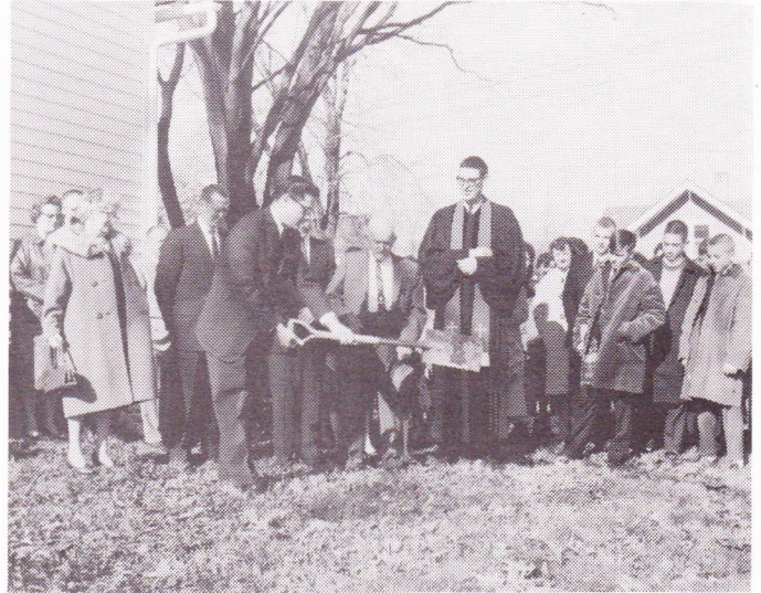
Ground breaking for the new education building in 1964. Don Potter with shovel with Aletha Weaver, Ervin Knox, Wm. Bryant and Rev. Ronald Byars looking on.
